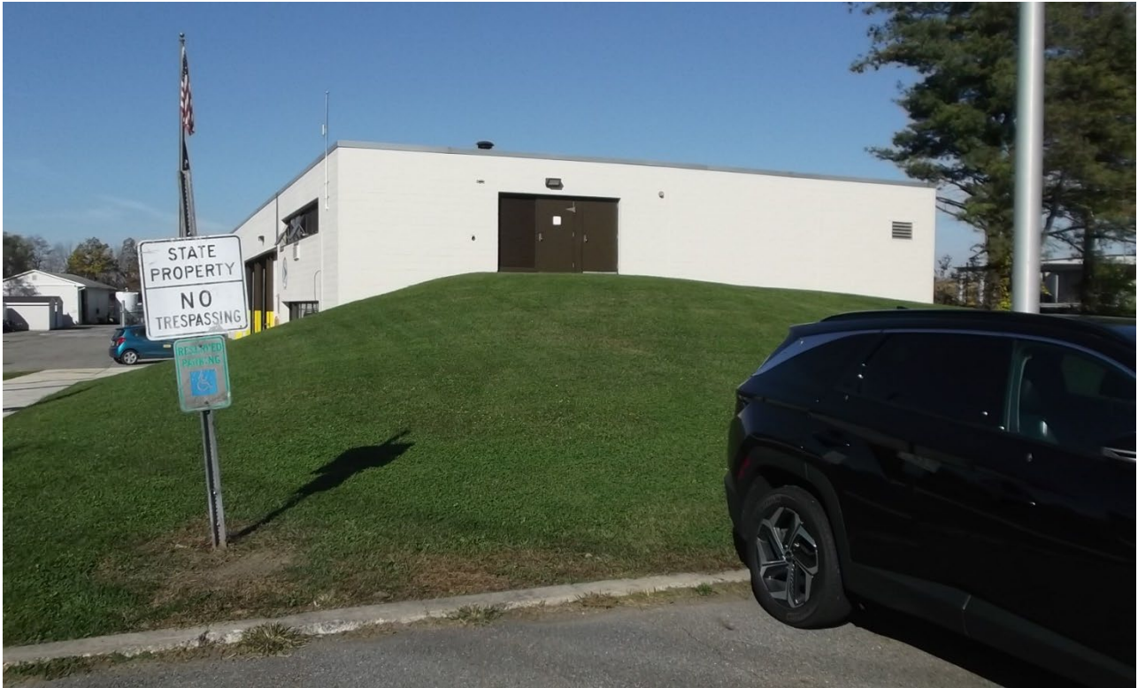
View of access door to mechanical room at DOT Lafayette Maintenance Facility.
