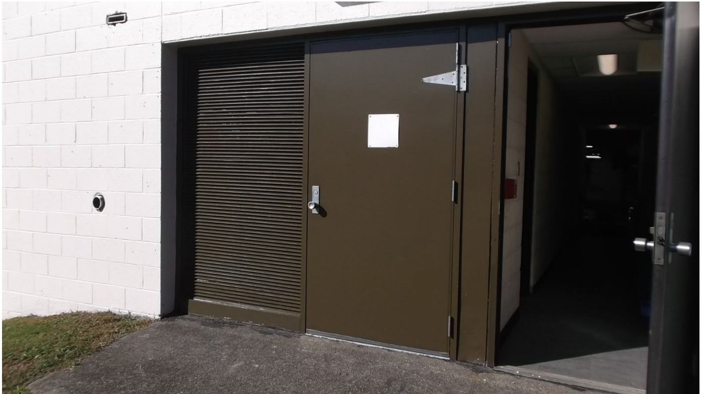
Mechanical room is on the left.
